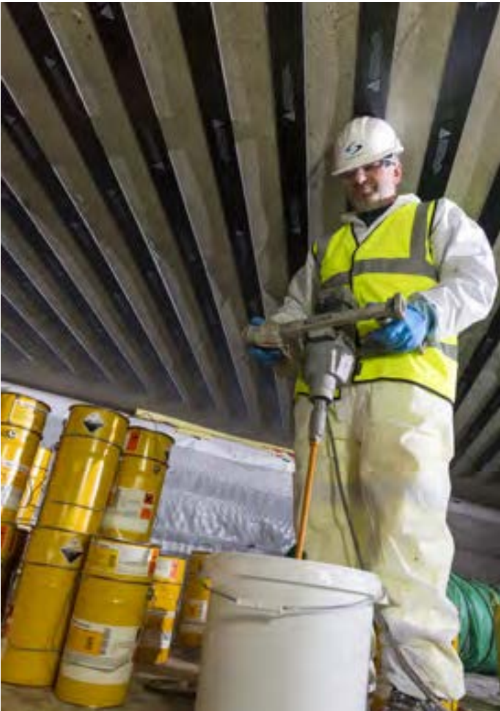
Application of Sikadur®-30 adhesive to carbon fibre plates.
