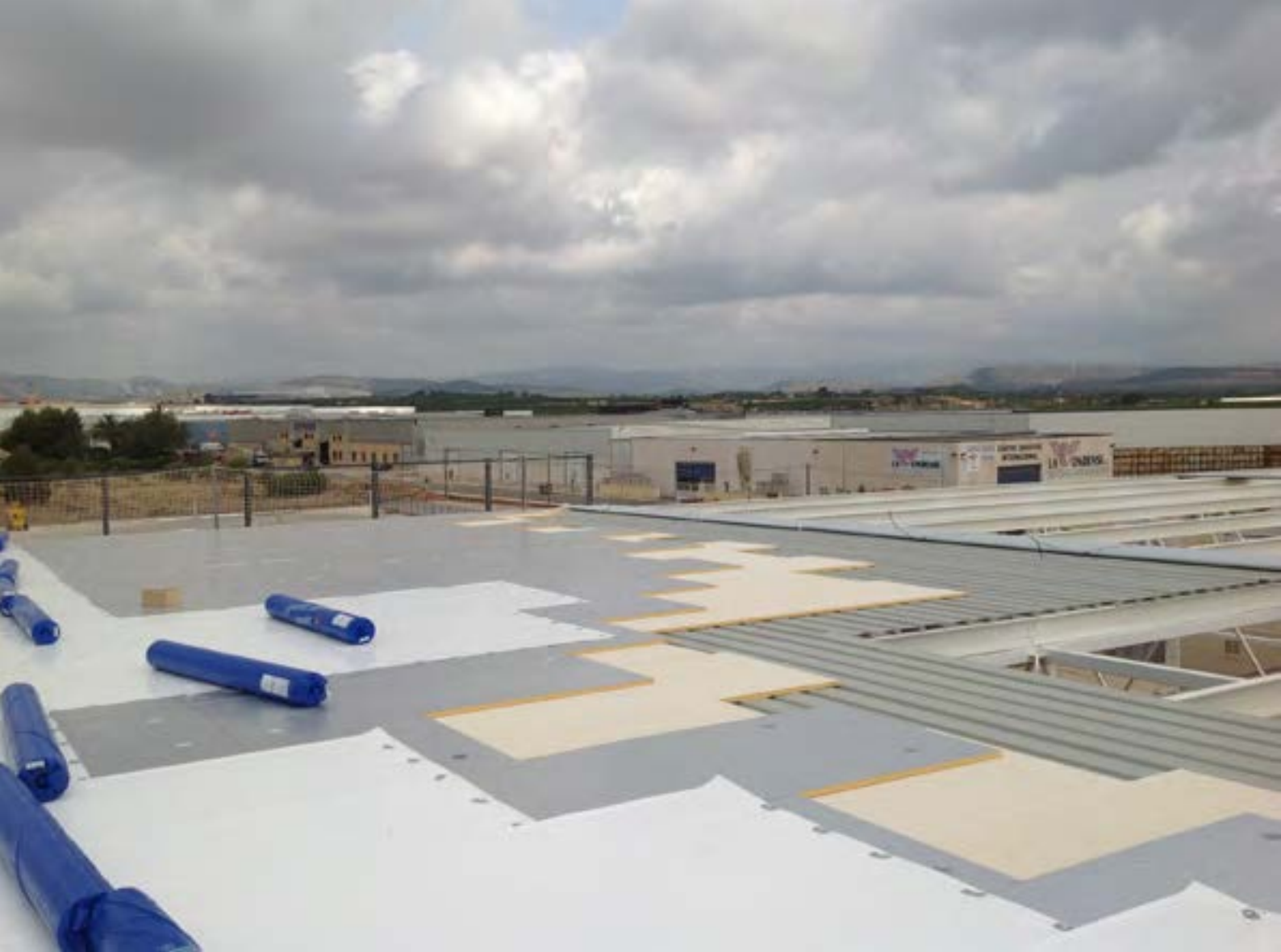
The results for a roofing system treated with beige Sarnafil TS 77-18 and one with white Sarnafil TS 77-18 SR demonstrate that both thermoplastic membranes bring significant savings.
