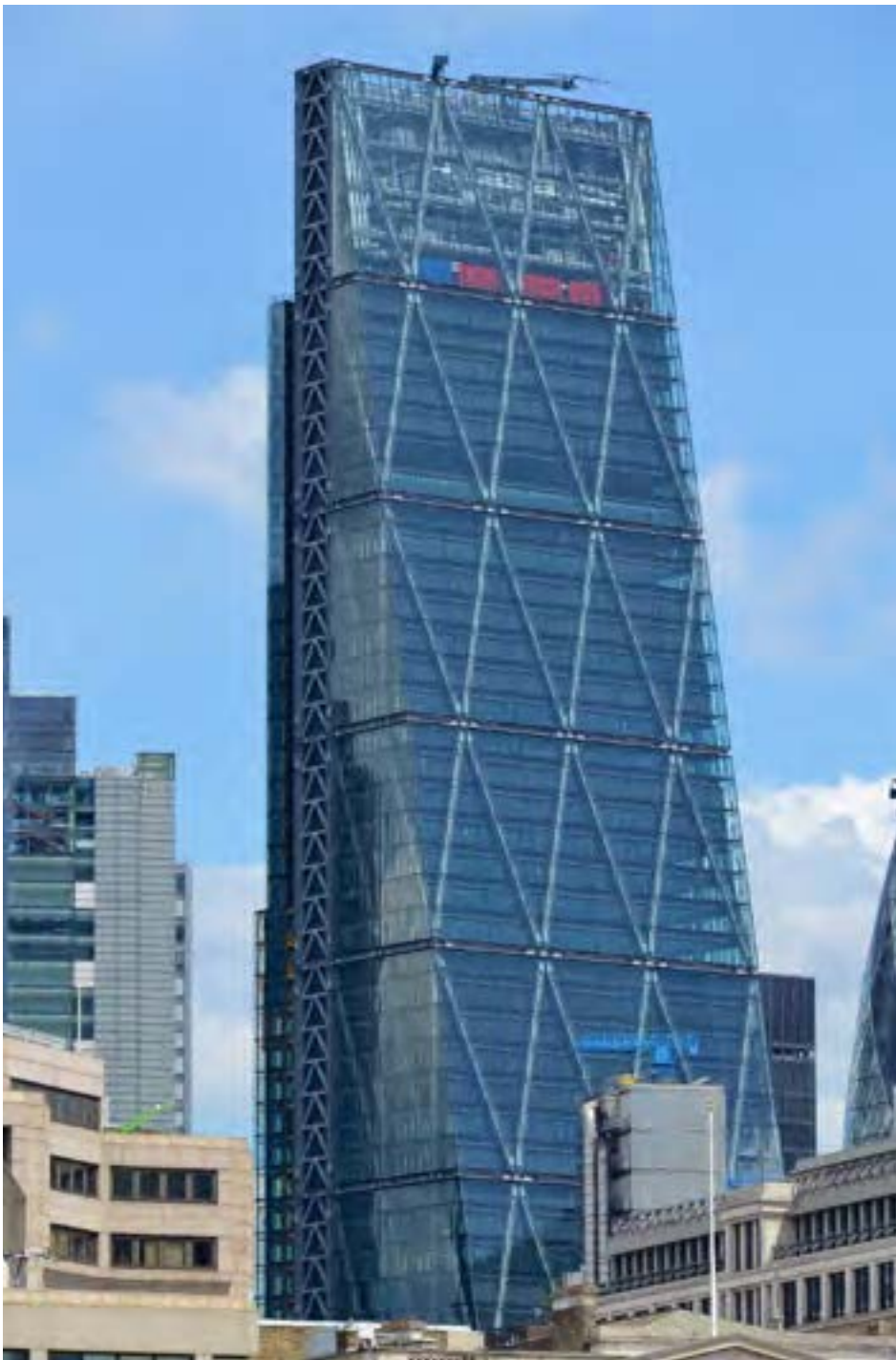
Designed by Richard Rogers and developed by British Land and Oxford Properties, the new Leadenhall Building will be 225 m tall, with 48 floors
