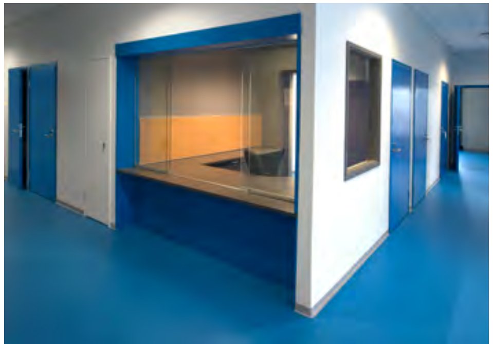
The walls in the washing and communal areas were treated with seamless Sikagard Hygienic coatings – a novel solution for Finland.
