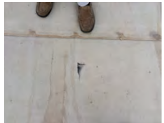
Cracks in the old roof.
