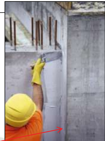
Sikadur Combiflex SG (Cinta impermeable flexible de poliolefina)
