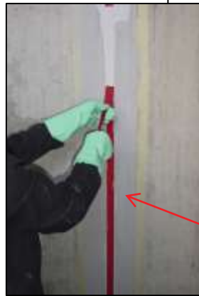
Sikadur Combiflex SG (Cinta impermeable flexible de poliolefina)
