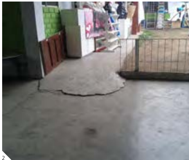
1. Sealing joints – Sikaflex®- 11 FC 2. Repairing cracks – Sikadur® and Sika Rep®
